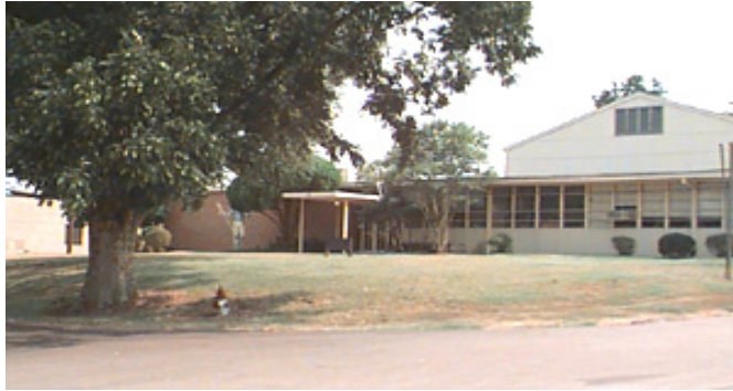
Figure 4: Front Entrance Alcorn ROTC Military Science Facility
